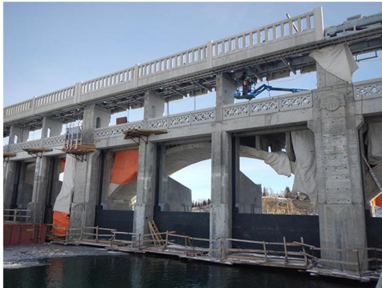
The gates are raised and lowered using a hoist. It will be powered electrically meaning the gates can be raised or lowered in a matter of minutes. The gates shown here are in the down position.
